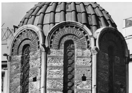
Figure 175 Kapnikarea. The dome of the church.
